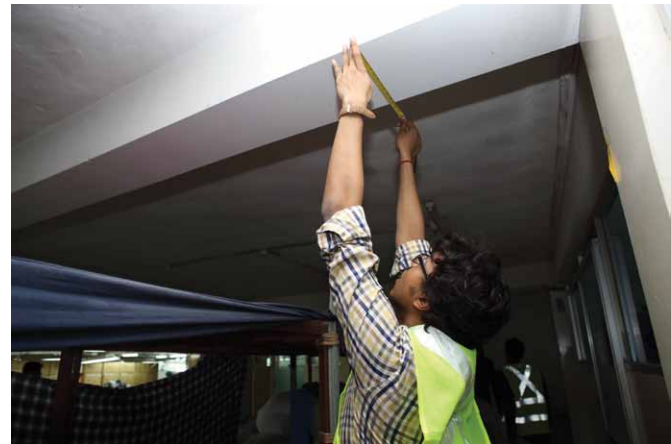
Following safety inspections, remediation work is now top priority in the RMG sector
